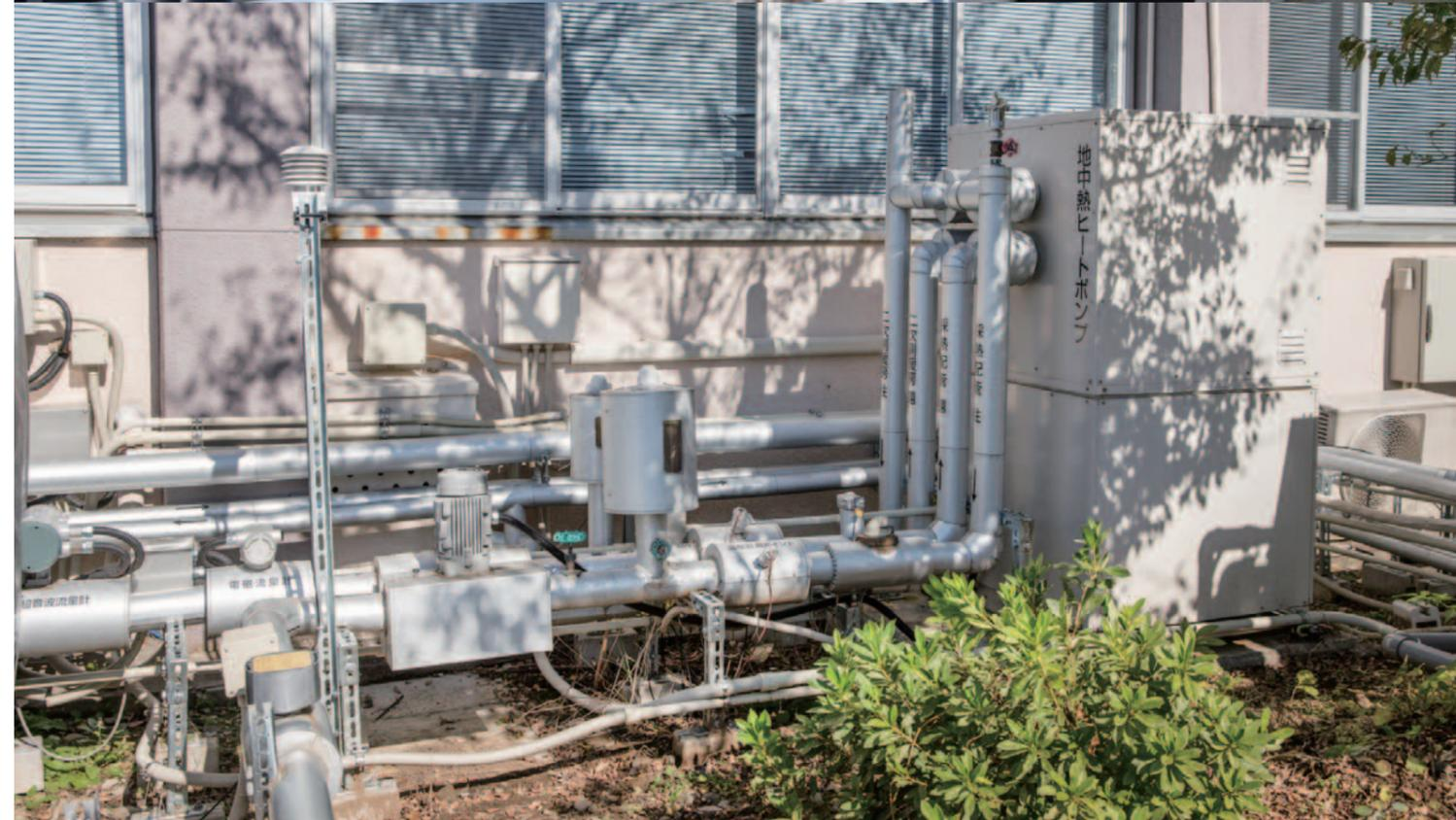
(Top photo) Professor Takeda explains ground heat data. (Bottom photo) Ground source heat pump installed next to the laboratory and actually used for air conditioning.
